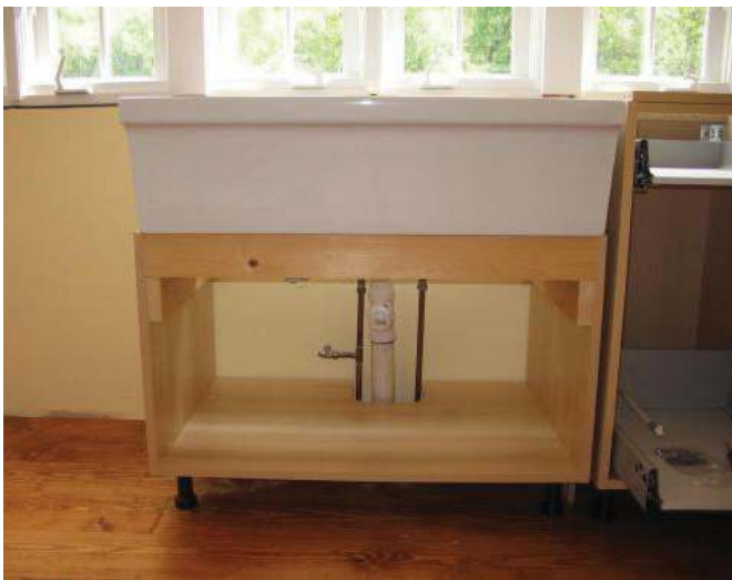
[Above]: Cabinet and sink in place.
