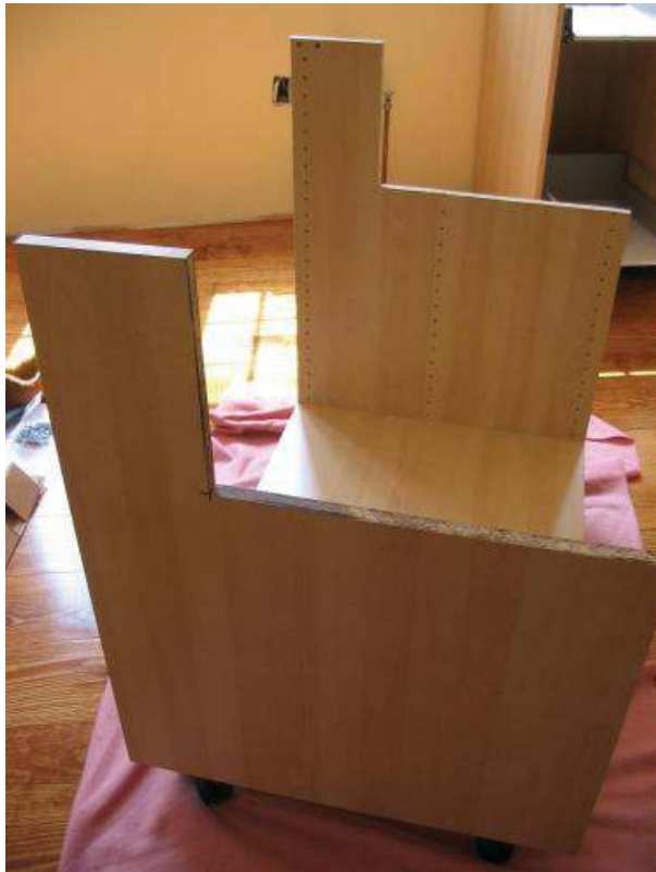
[Above]: After making the cuts, the cabinet is ready to be assembled.
