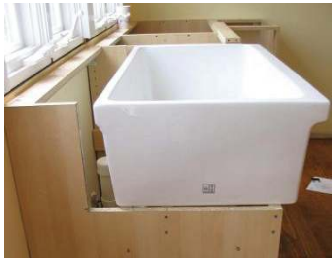
[Above]: Checking clearance on all sides of the sink.
