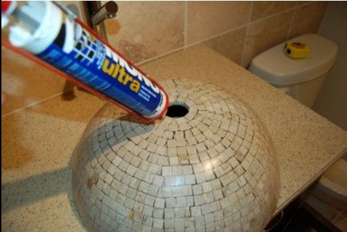
Above: Process for "Above Counter Mounting"
