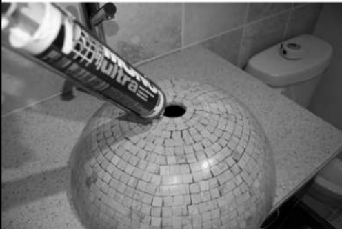
Above: Process for "Above Counter Mounting"
