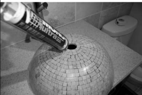
Above: Process for "Above Counter Mounting"
