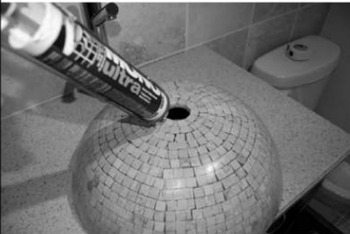
Above: Process for "Above Counter Mounting"
