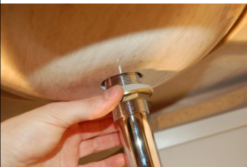
Above: Drain Attachment
